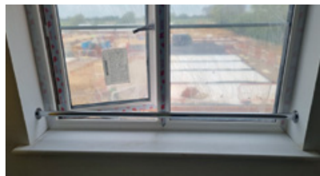
Figure 1: Example of a Part O compliant guard rail
